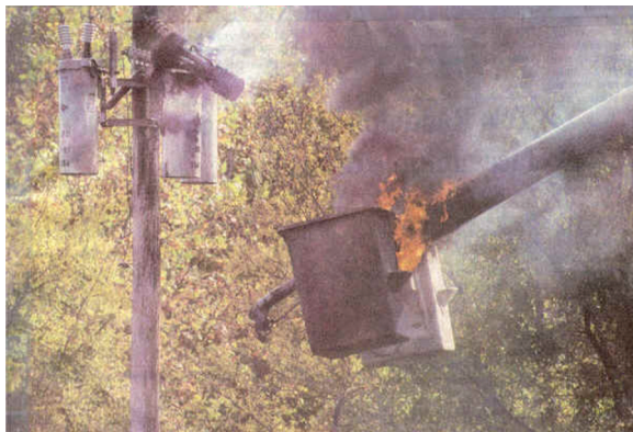
Figure 8.35 Explosion of a recloser that caused a fatality. (From Dalton Sullivan, Pocahontas (AR) Star Herald. With permission.)
