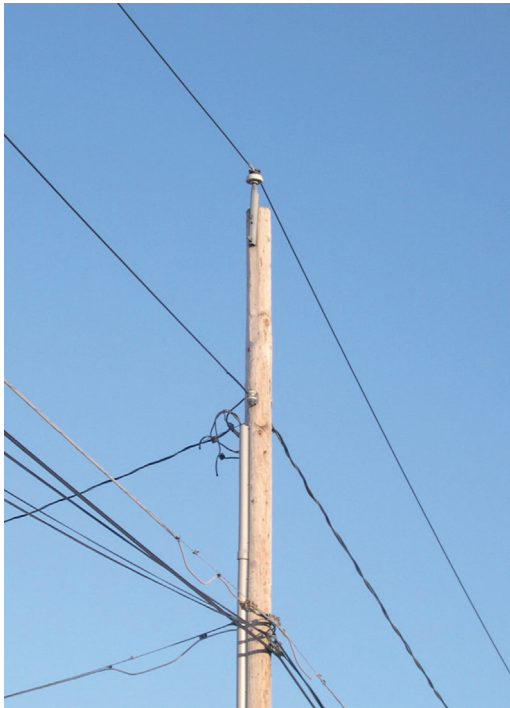
Figure 2.2 Single-phase circuit, 7.2 kV line-to-ground.
