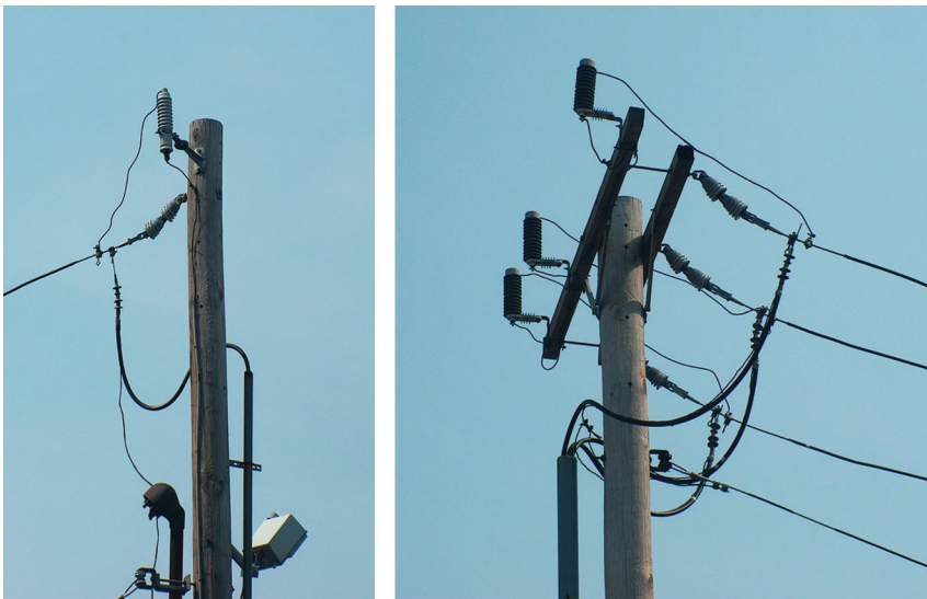
Figure 13.21 Arrester applications with long lead lengths.
