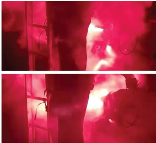
Figure 14.41 Infrared filtered video frames of an EPR splice failure. (From EPRI 1018693, Distribution Arc Flash: Analysis Methods and Arc Characteristics , Electric Power Research Institute, Palo Alto, CA, 2009. Copyright 2009. Reprinted with permission.)
