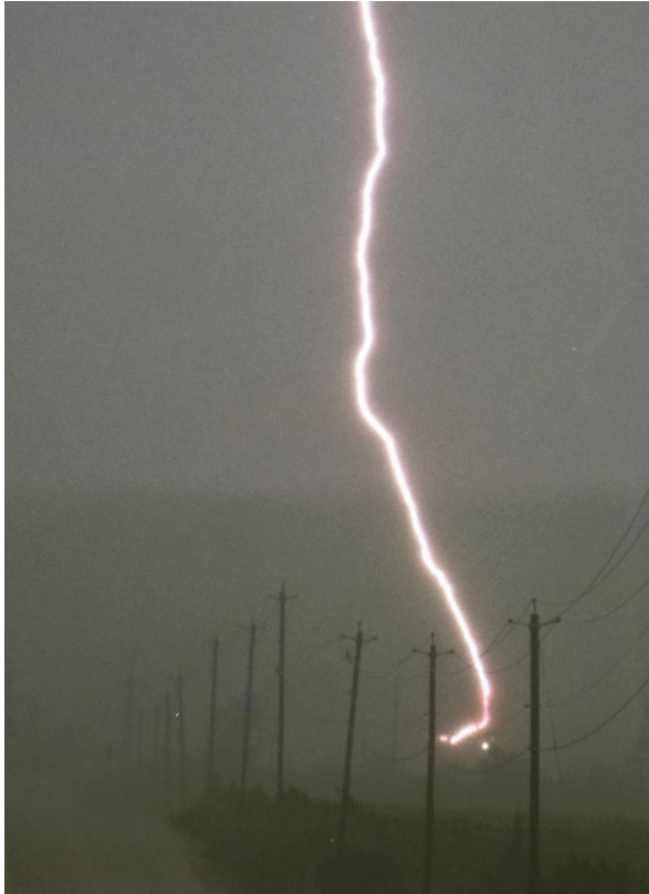
Figure 13.16 Lightning flash that failed an arrester. The circuit in the foreground curves around to the right about a mile beyond the visible poles. Flashovers occurred at poles on either side of the strike point. An arrester failed on one of the poles. (From Niagara Mohawk Power Corporation. Copyright 1991. Reprinted with permission.)
