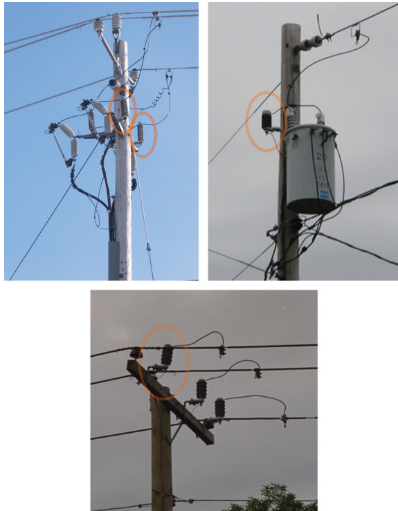
Figure 13.12 Example of arrester applications.
