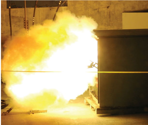
Figure 14.39 Example arc flash in a medium-voltage padmounted switch. (From EPRI 1022697, Distribution Arc Flash: Phase II Test Results and Analysis , Electric Power Research Institute, Palo Alto, CA, 2011. Copyright 2011. Reprinted with permission.)
