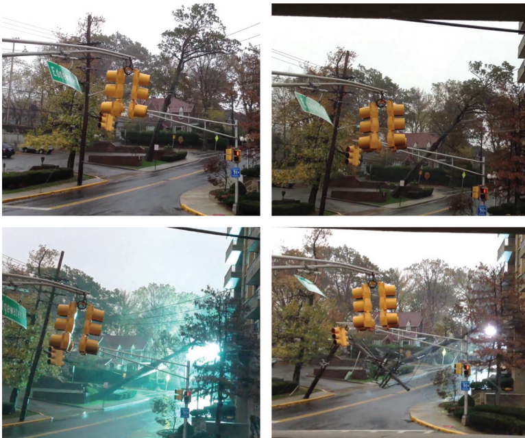
Figure 3.1 Video sequence of a falling tree causing a fault and breaking a pole. (Courtesy of Alexander Kirichenko. http://youtu.be/-gUD31Bqnuo .)
