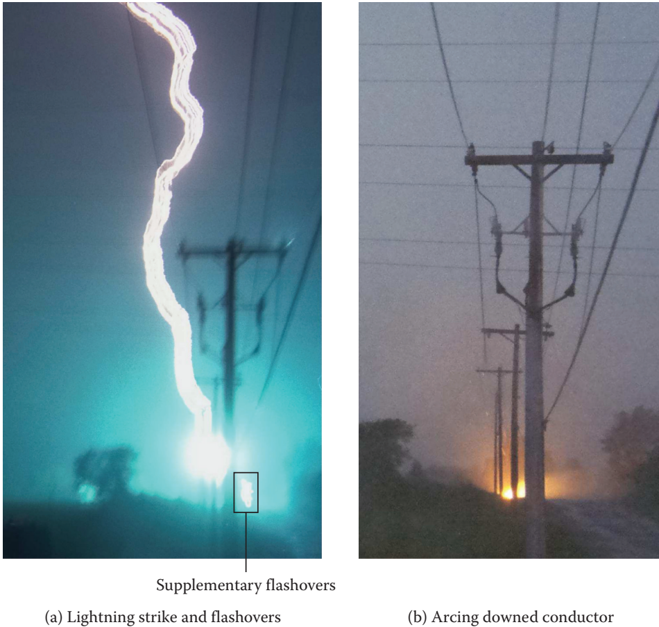
Figure 13.1 Example of a lightning flash to a 13.2-kV distribution line and the downed wire that resulted. (From Niagara Mohawk Power Corporation. Copyright 1991. Reprinted with permission.)
