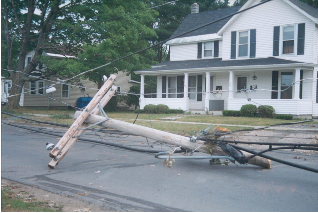
Figure 3.29 Example of a pole broken by a tree in a large wind storm.
