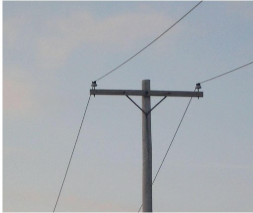
Figure 2.3 Single-phase, 4.8-kV circuit.
